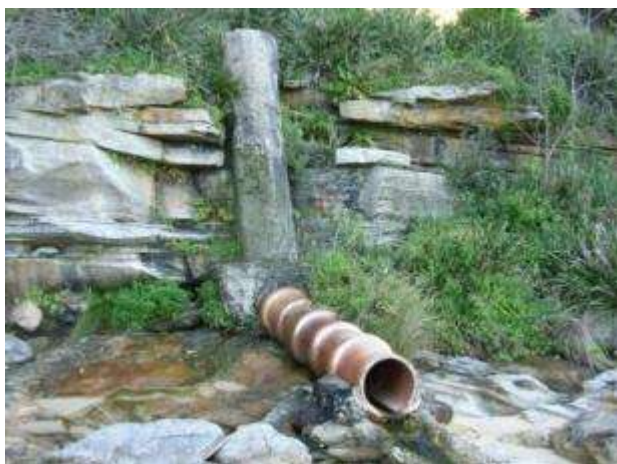
Fig 6.5e: Stormwater outlet on top of rock outcrop on Delwood beach further east.
