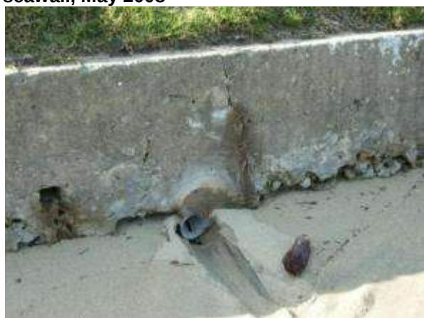
Fig 5.16.1a: Drainage provision in the Fairlight seawall, May 2008
