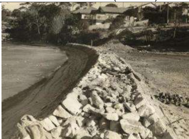
Construction of outfall drain (22.07.1938)
