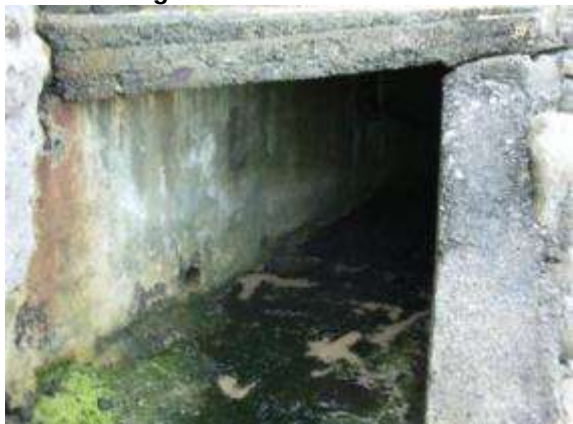
Fig 6.5a: Stormwater box culvert at western end of Fairlight beach
