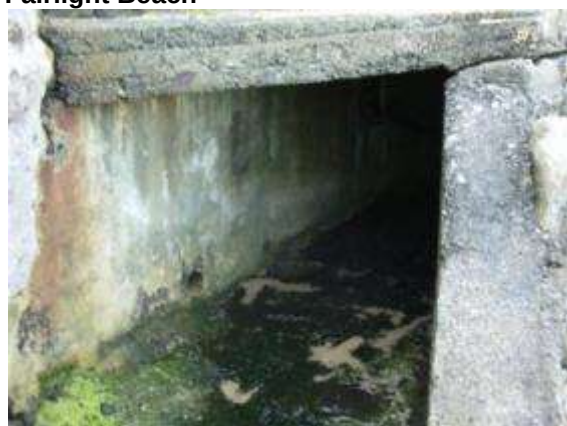
Fig 5.16.1b: Drainage culvert at western end of Fairlight Beach
